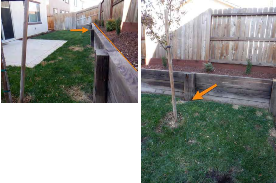
Wood Deterioration
