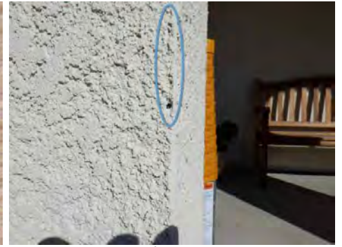
Facing Front Porch
