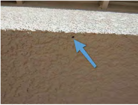
Right of Garage Door, Under Eaves
